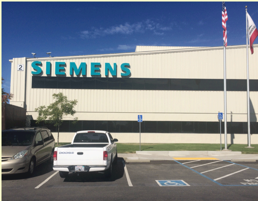
Florin Facility Front (photo by G. Huckaby)
