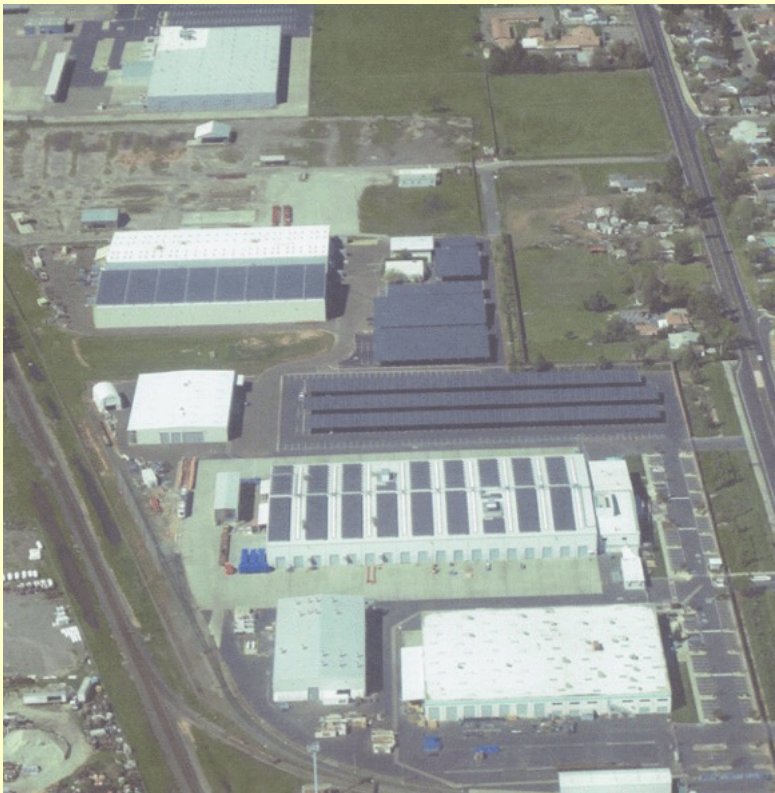
Aerial View of Siemens' Florin Facility (photo courtesy of Siemens Publicity)
